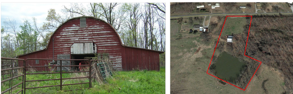
Figure 23: BA-180, NRHP-eligible barrel-vault mule barn
